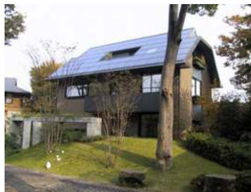
Roof integrated PV in Japan
